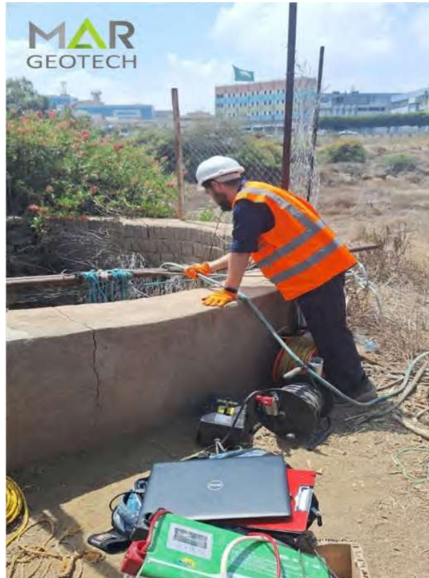
Hydrology Survey - Abaha
