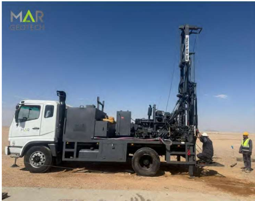
Truck Mounted Drilling Rig-04
