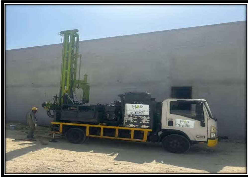
Truck Mounted Drilling Rig -01
