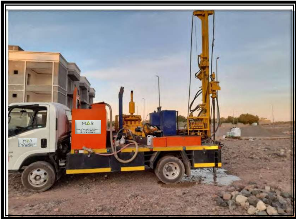
Truck Mounted Drilling Rig -03
