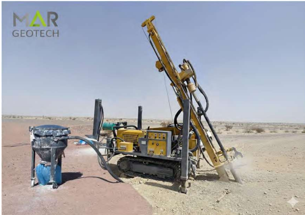
Track Mounted Drilling Machine
