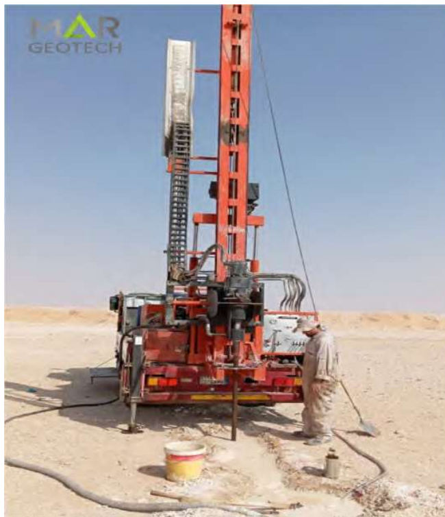
Truck Mounted Drilling Rig-05
